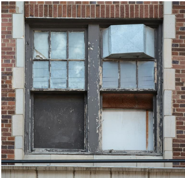
ORIGINAL DOUBLE HUNG WINDOW NOT BEING REPLACED
