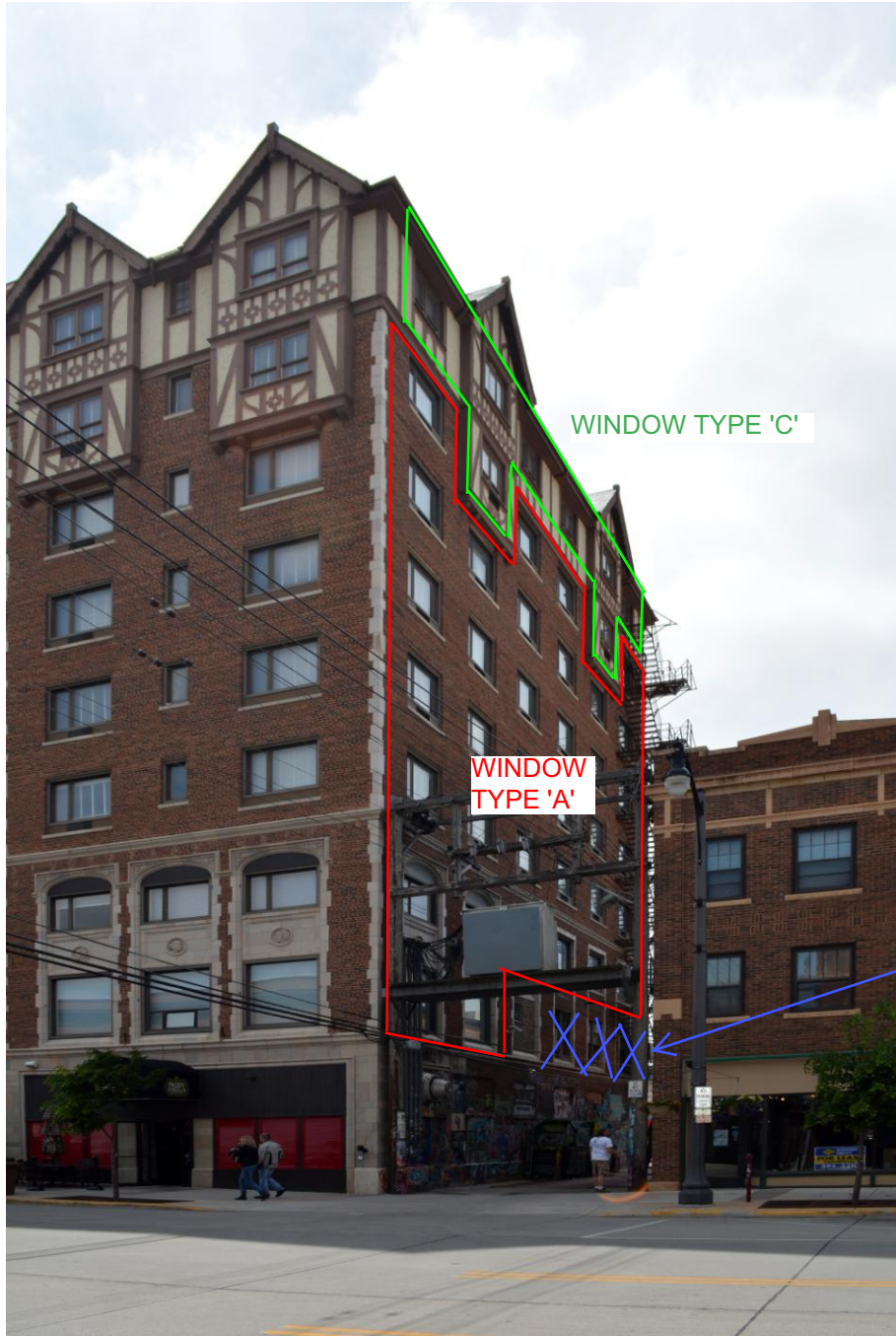
NORTH SIDE OF BUILDING (ALLEY SIDE)
